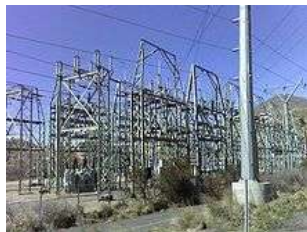
Electric Power Distribution
